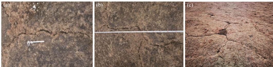
Fig. 2 Developmental morphological of surface cracks in alpine meadows. (a), linear fracture; (b), dendritic fracture; (c), polygonal fracture.
